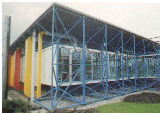
*Facade Detail Bridge to the old office building View
